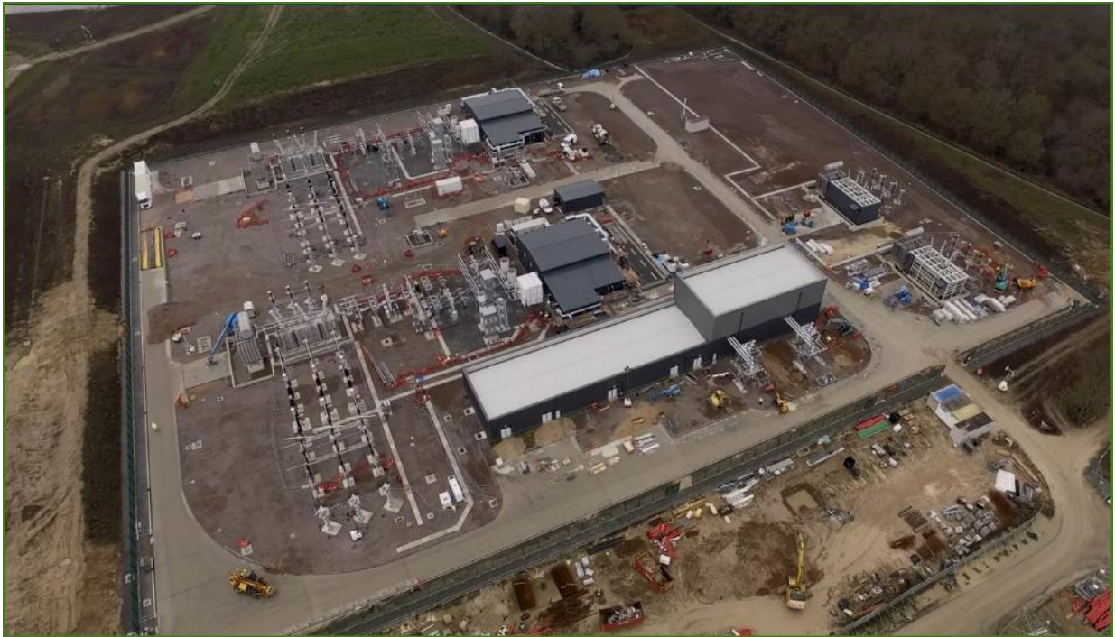
Plate 6.1 Example Layout of the Onshore Substation (example taken from construction of East Anglia ONE substation)
